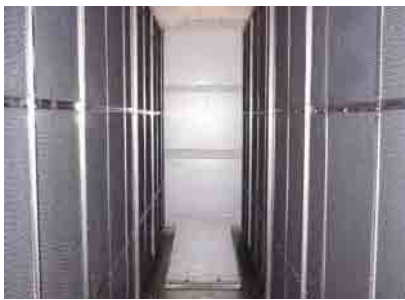
Water-curtain external-air treatment air conditioner
