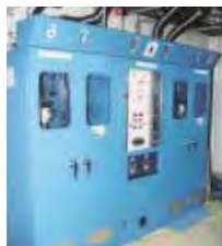
The cylinder cabinet is equipped with multiple sensors
