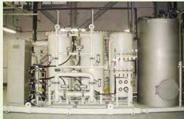
Organic sludge reduction system
