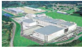
Panoramic view of the Kameyama Plant
