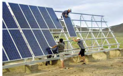
Banks of photovoltaic modules being installed
