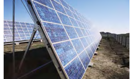
Brilliant sunshine falls on completed photovoltaic modules
