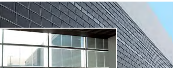
Crystalline, thin-film, see-through photovoltaic modules installed on the wall of Plant No. 2
