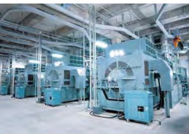
A cogeneration system produces about one-third of the electricity used in the whole plant
