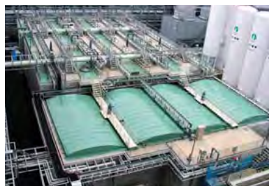
Drainage facilities recycle all process wastewater
