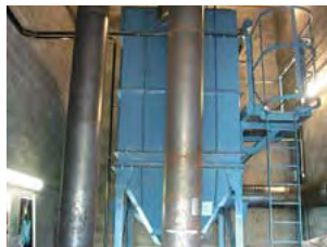
Introduction of a vacuum dust collector
