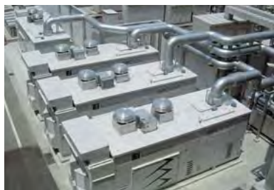
A 1,000-kW fuel cell system, Japan's largest
