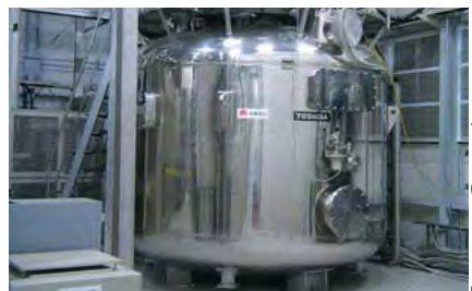
A 10-MVA superconducting magnetic energy storage system supplies electricity in case of sudden drops in voltage
