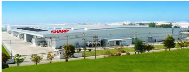
SATL's new Cool e 3 plant
