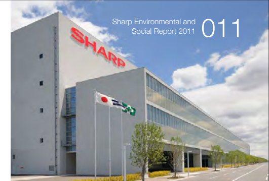
Solar cell plant at GREEN FRONT SAKAI
