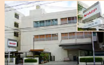
The current office building
