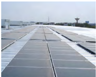
Solar power generation system
