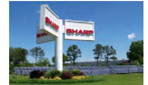
Solar array on SMCA premises
