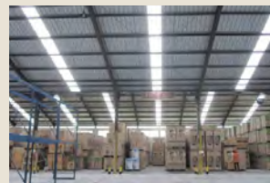
Roofing that lets in natural light
