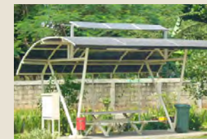
Solar power system installed on plant grounds
