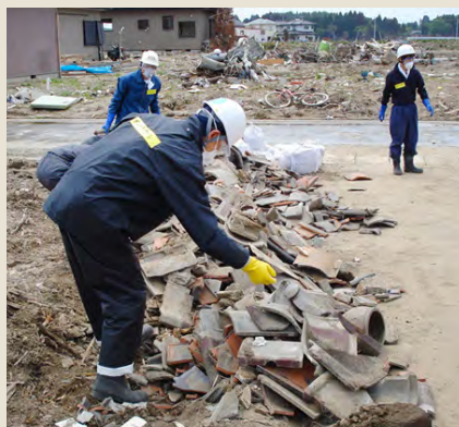
Volunteer reconstruction activities by employees
