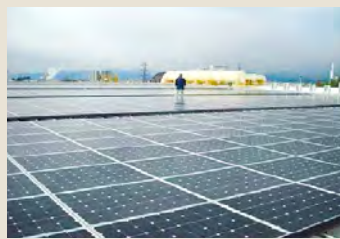
Solar power system installed on the roof of KRSC's main plant
