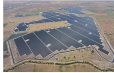
Mega-solar power plant in Thailand
