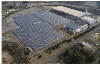
Sharp Daisen no Mori Solar Power Plant (Yonago, Tottori Prefecture, Japan)
