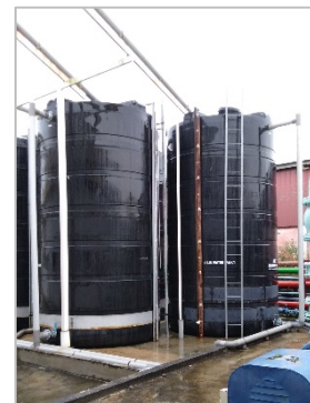
Rainwater tanks installed in the plant
