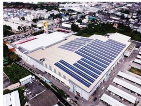
Installation of rooftop solar modules
