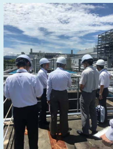
RBA auditor (third from left) checks factory wastewater treatment equipment together with Sharp personnel
