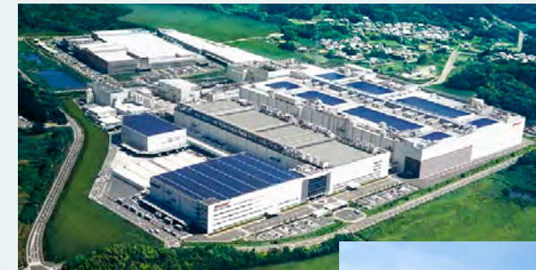
5,210 kW solar power generation system installed on the roof and walls at the plant
