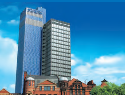
CIS Tower, Manchester, UK
