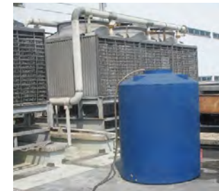
Reducing the factory's environmental impact by installing water recycling equipment on the cooling tower
