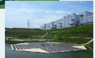
Floating 200 kW solar power generation system set up in cooperation with Kameyama City on a stormwater retention pond that is adjacent to the factory. Proof-of-concept tests are underway.
