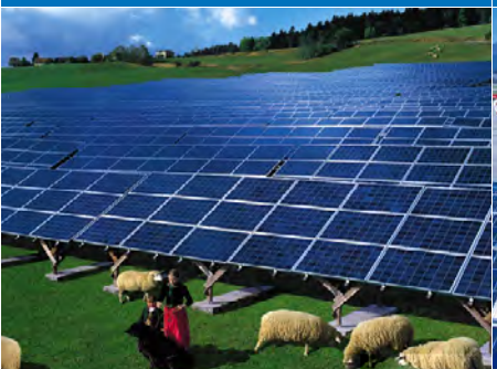
Solar power plant, Sonnen, Bavaria, Germany
