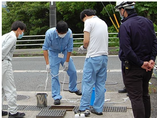
Wastewater sampling and analyses by three parties
