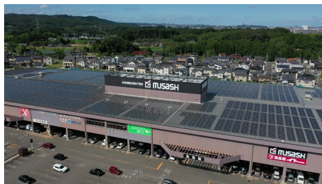
Industrial solar power system
