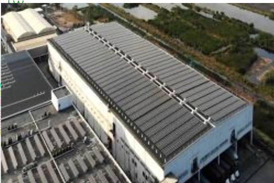
■ New solar rooftop system at Warehouse-1 ; 1,634.04 kW
